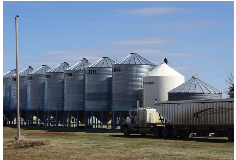
Grain bins located under overhead lines are a serious safety concern, and encroach on SaskPower's right-of-way, which landowners are required to keep clear.
